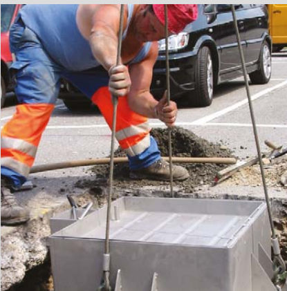
Adapting the unit and levelling onto the correct installation depth (lining surface level).
