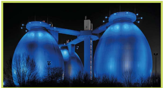
DeltaLUXX Blue - Outdoor sewage treatment plant lighting
