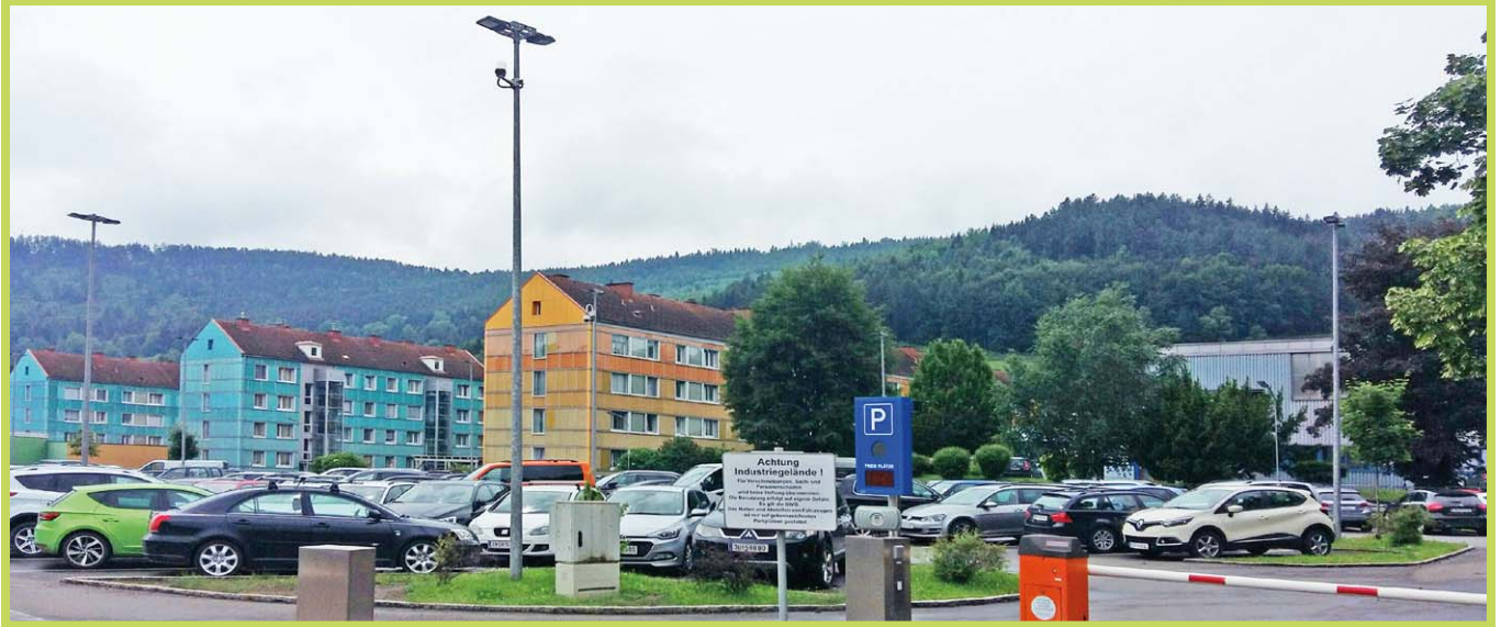
PLAZA FlatLED - Parking lot lighting
