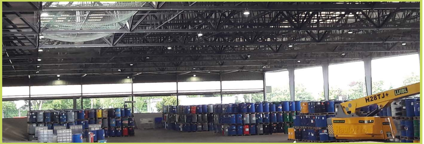
DeltaLUXX - Storage space lighting
