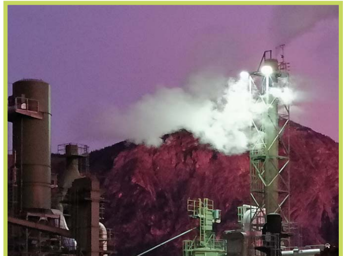
High Power LED - Illumination of factory premises
