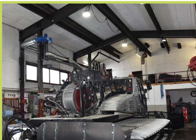
DeltaLUXX - Snow grooming workshop lighting
