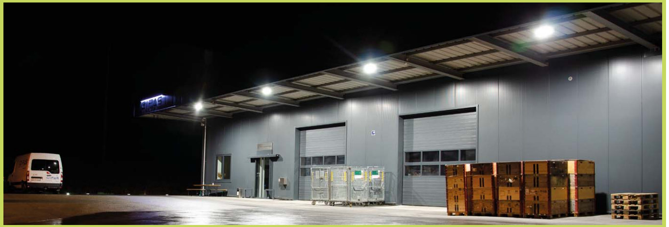
AlphaLUXX - lighting of warehouses / storage areas
