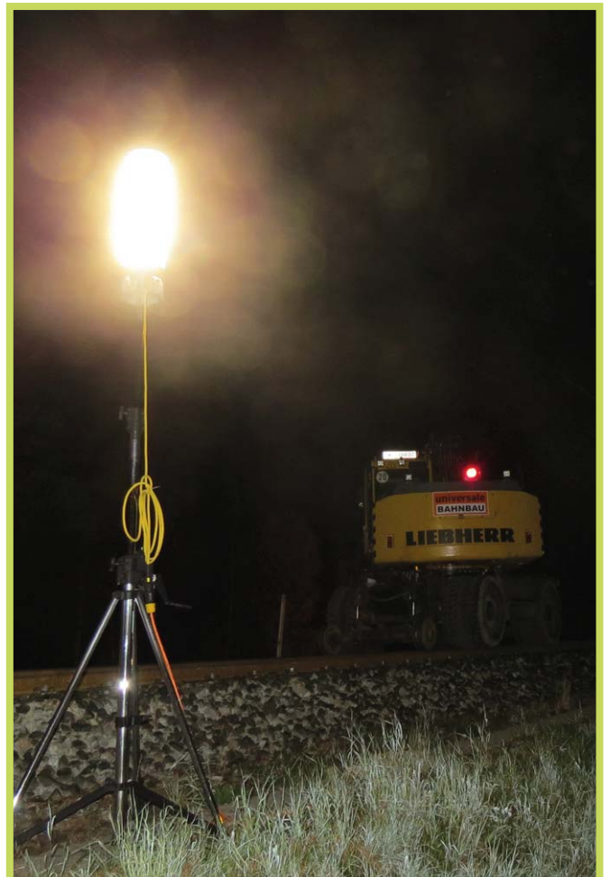
ApolloLED - Construction site use
