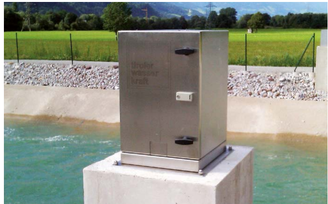
Stainless steel socket distributor - TIWAG Jenbach
