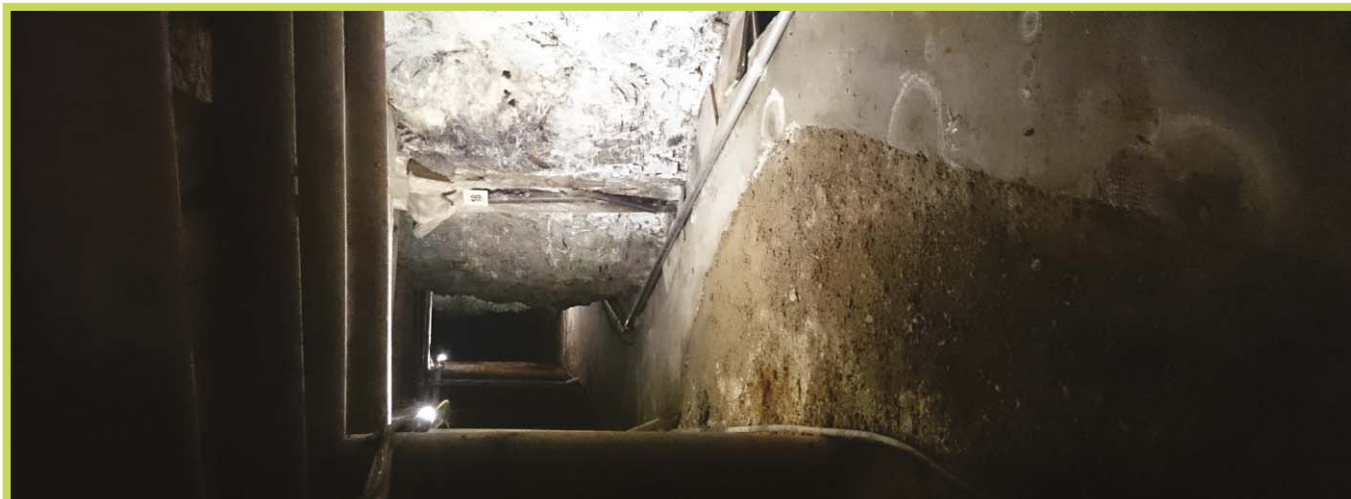
StreamLED Power - Osvetlenie v tuneli
