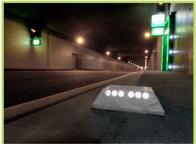
Tunnel St. Maurice, Wallis
