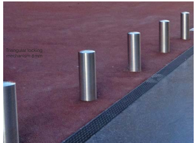
Fixed bollard Wien
