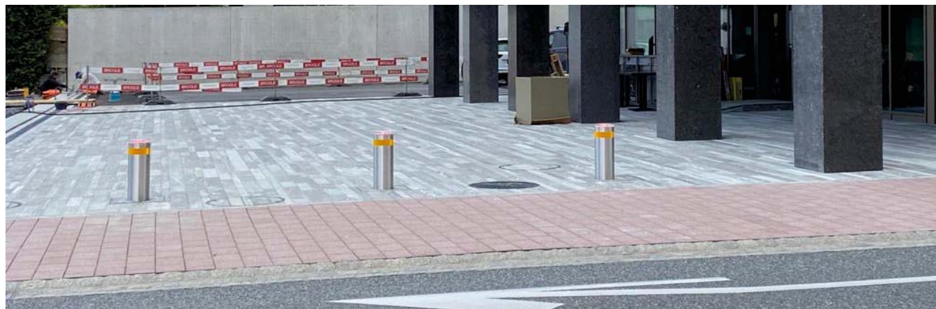
3x Retractable bollards 2.0, Office building
