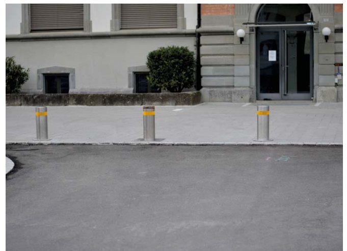
Fixed bollards and Retractable bollard school Thal
